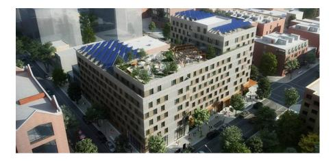
Throops Corners, an all-electric multifamily building planned for construction in Brooklyn's Broadway Triangle, will provide 140 units of housing to low-income New Yorkers. The project will include solar power and be built to Passive House Standards.
